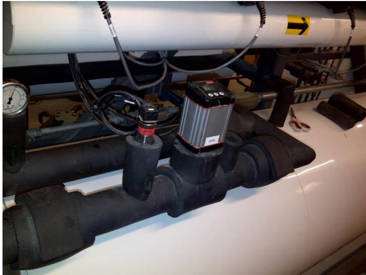
High-Pressure Expansion Valve
