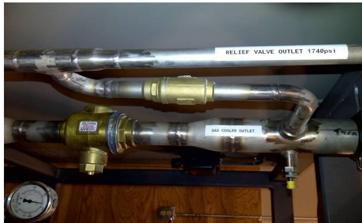
Pressure Relief Valve Piping
