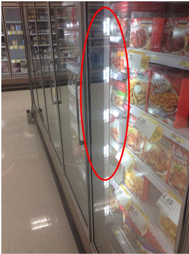
Installed wrong direction
