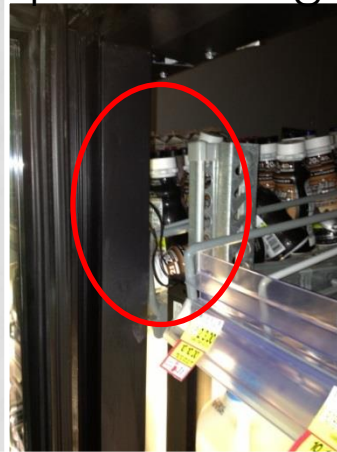
Exposed wiring
